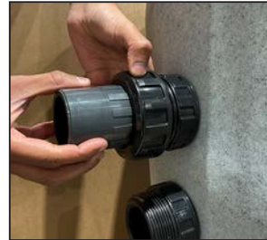
Screw the collar onto the outlet. HAND TIGHTEN ONLY.
