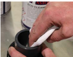
Clean pipe first
