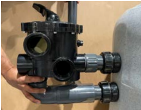
“Dry fit” pipework first
